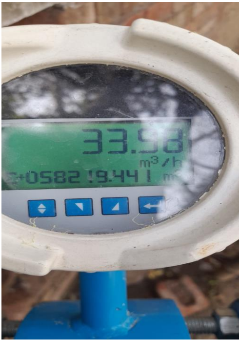
Water meter to measure the Volume of water at Water Treatment Plant
