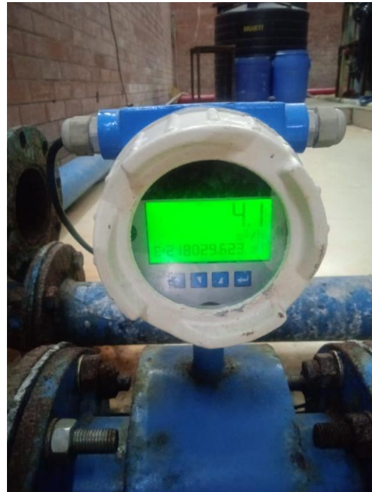
Water meter to measure the Volume of water at Water Treatment Plant
